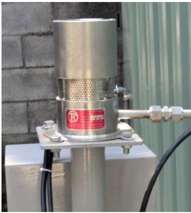
End of Line Flame Arrester, with Automatic Flare, was developed by RESI for Laboratory Applications.
